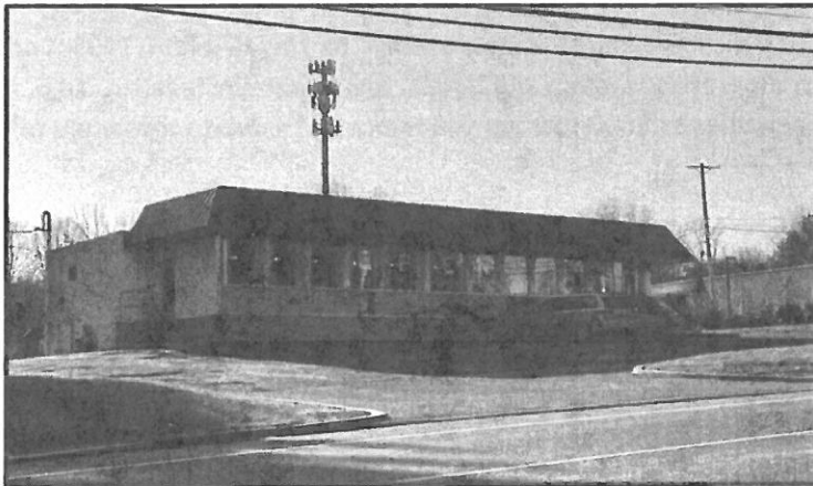
View of Amwell Valley Diner from Route 31 N.
