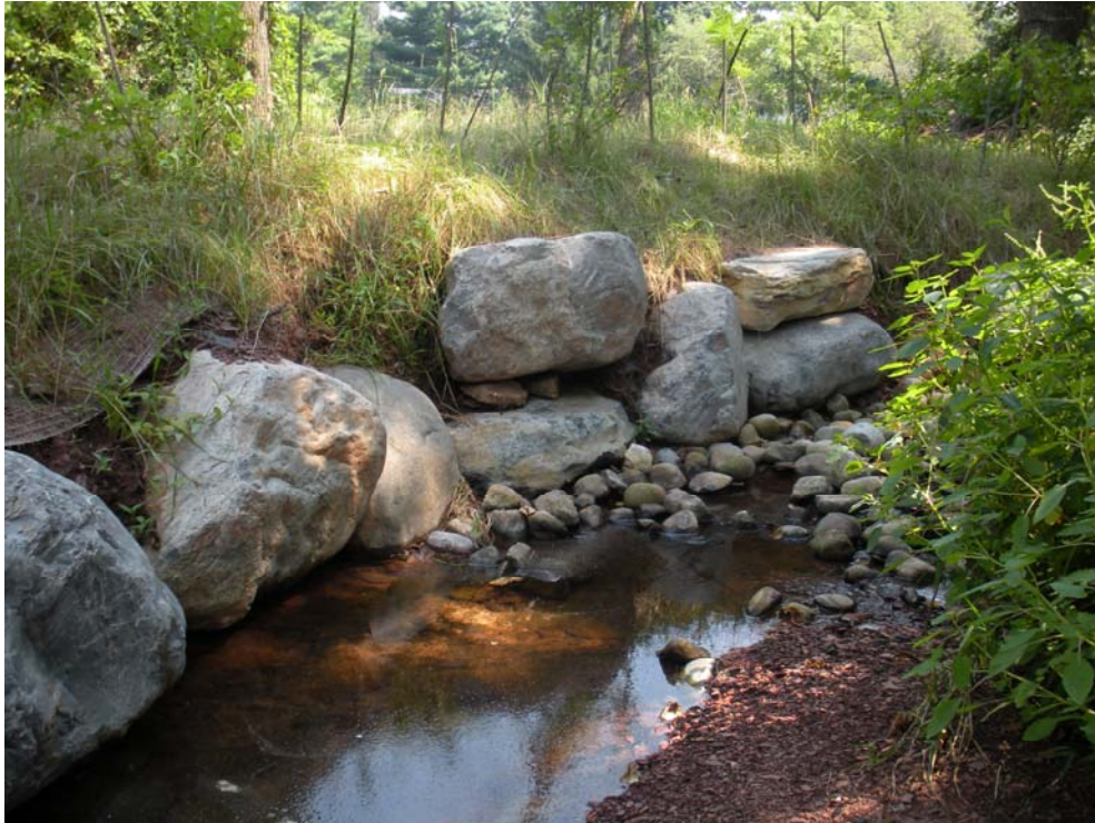
Figure 44: Boulder Toe Protection
