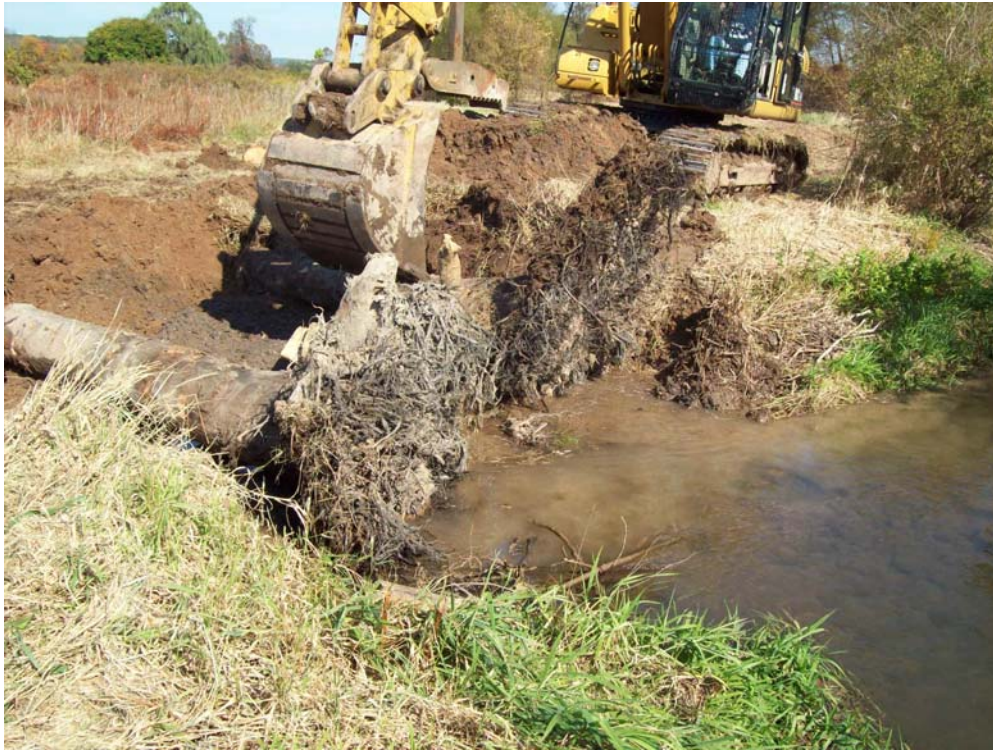
Figure 43: Rootwad Placement
