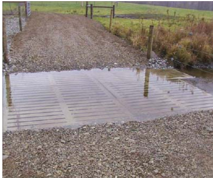
Figure 55: Improved Agricultural Stream Crossing
